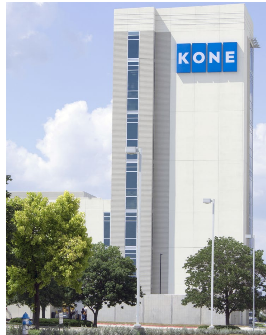
KONE's new facility in Allen, Texas features a test tower for evaluating prototypes and new components before they go into production.
