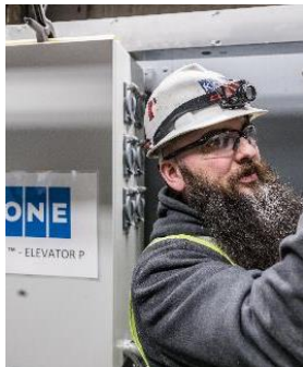
2001 KONE JumpLift construction time elevator
