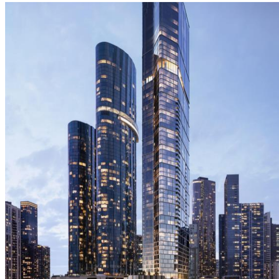
Melbourne Square BLVD, Australia
